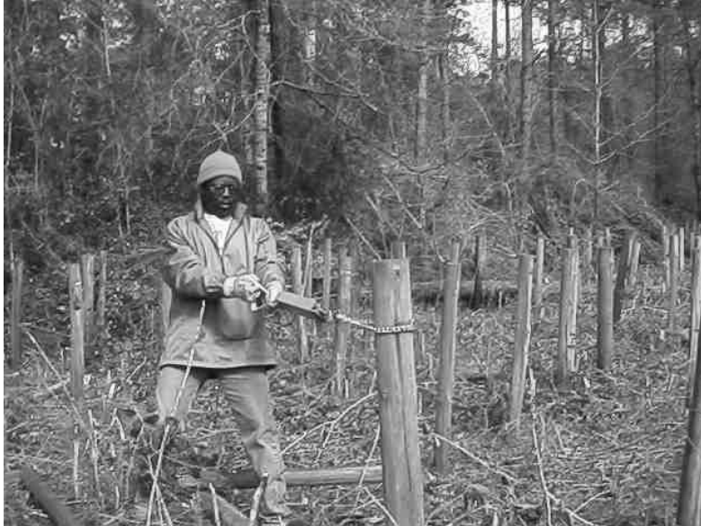
Example of 50 lb Pull test
